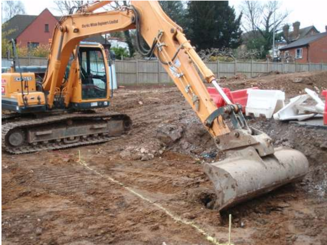
Plate 4. View of ground reduction (looking north-west)
